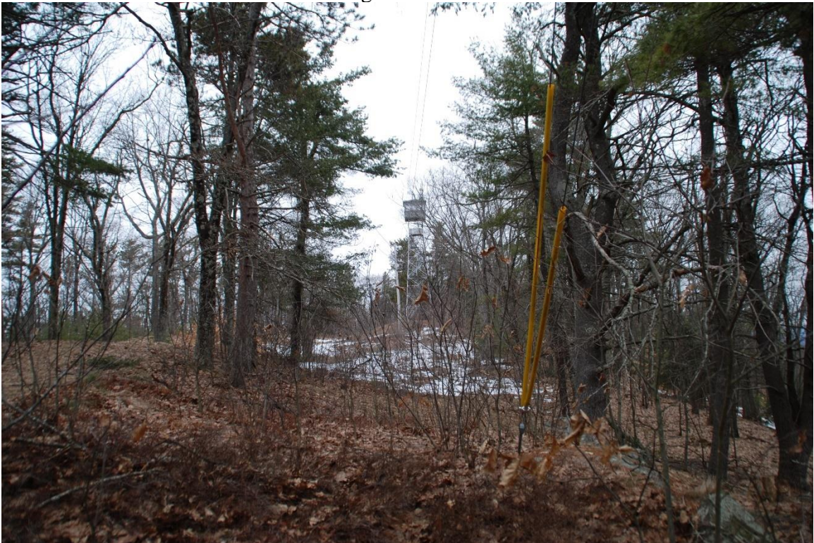
Photo 4. View north from the utility building along the overhead utility line.
