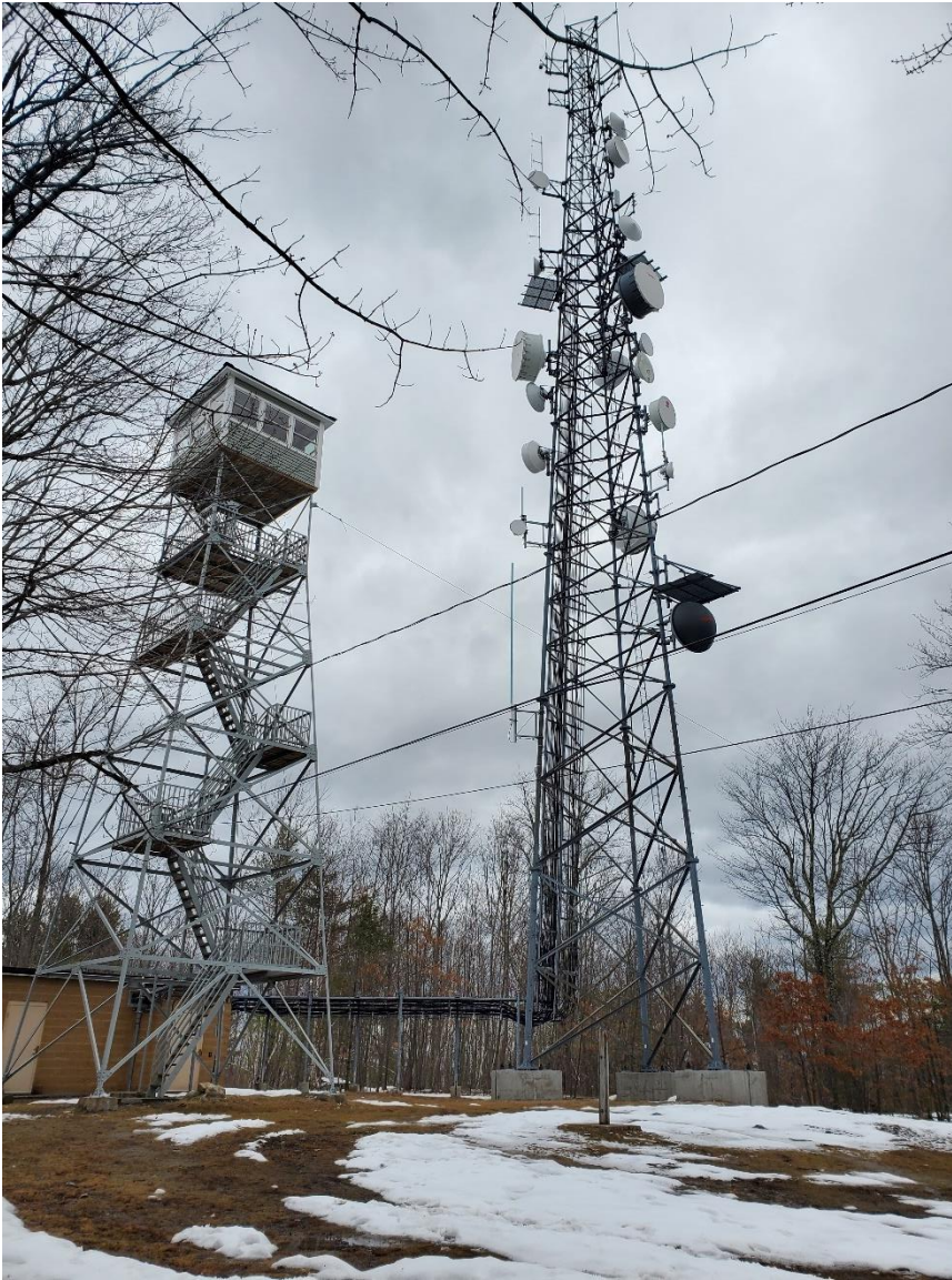
Photo 11. View northeast of the Oak Hill Fire Tower in Loudon, NH (LOU-0410), with the lattice telecommunication tower located within 50-ft.
