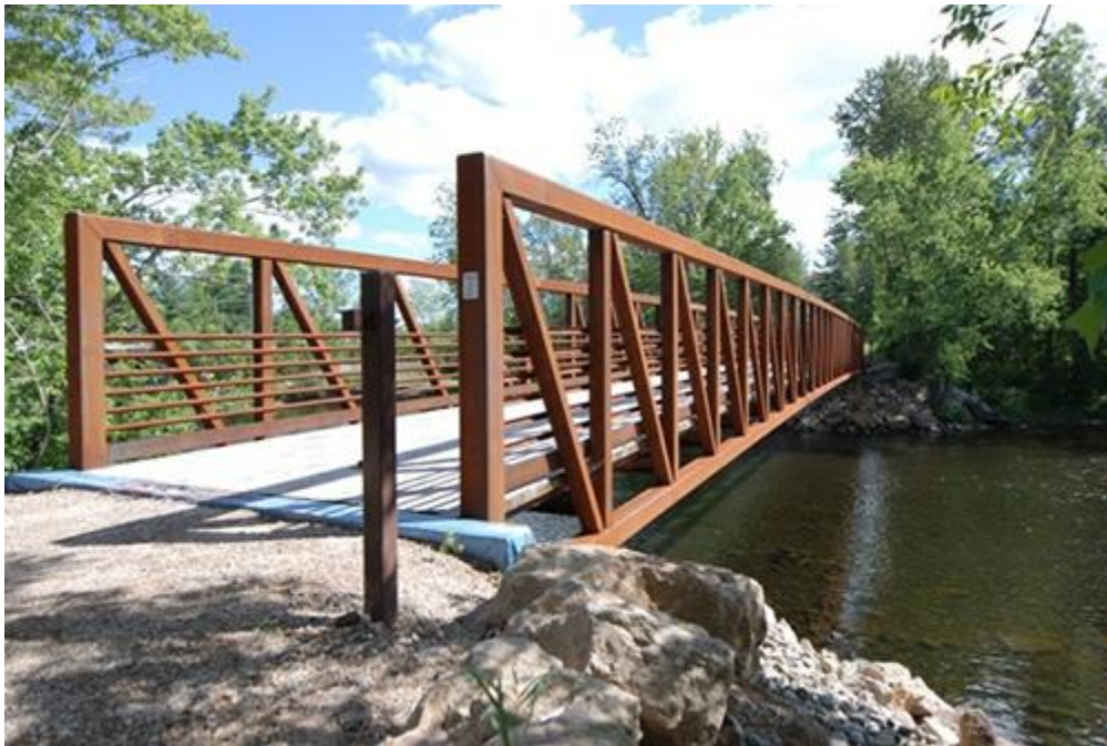
Pedestrian walkway bridge
