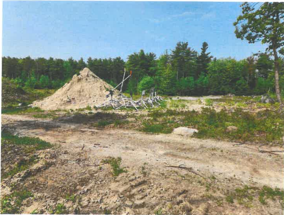
Looking west at existing dirt access road and temporary stockpiles.
