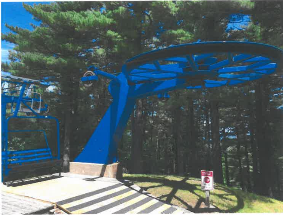
Looking northeast at the existing Hurricane Chair Lift unloading area.
