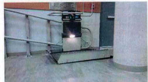
Modernization includes a new platform conveyance as shown
