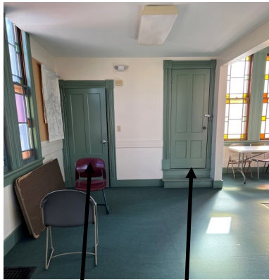
To basement attic
