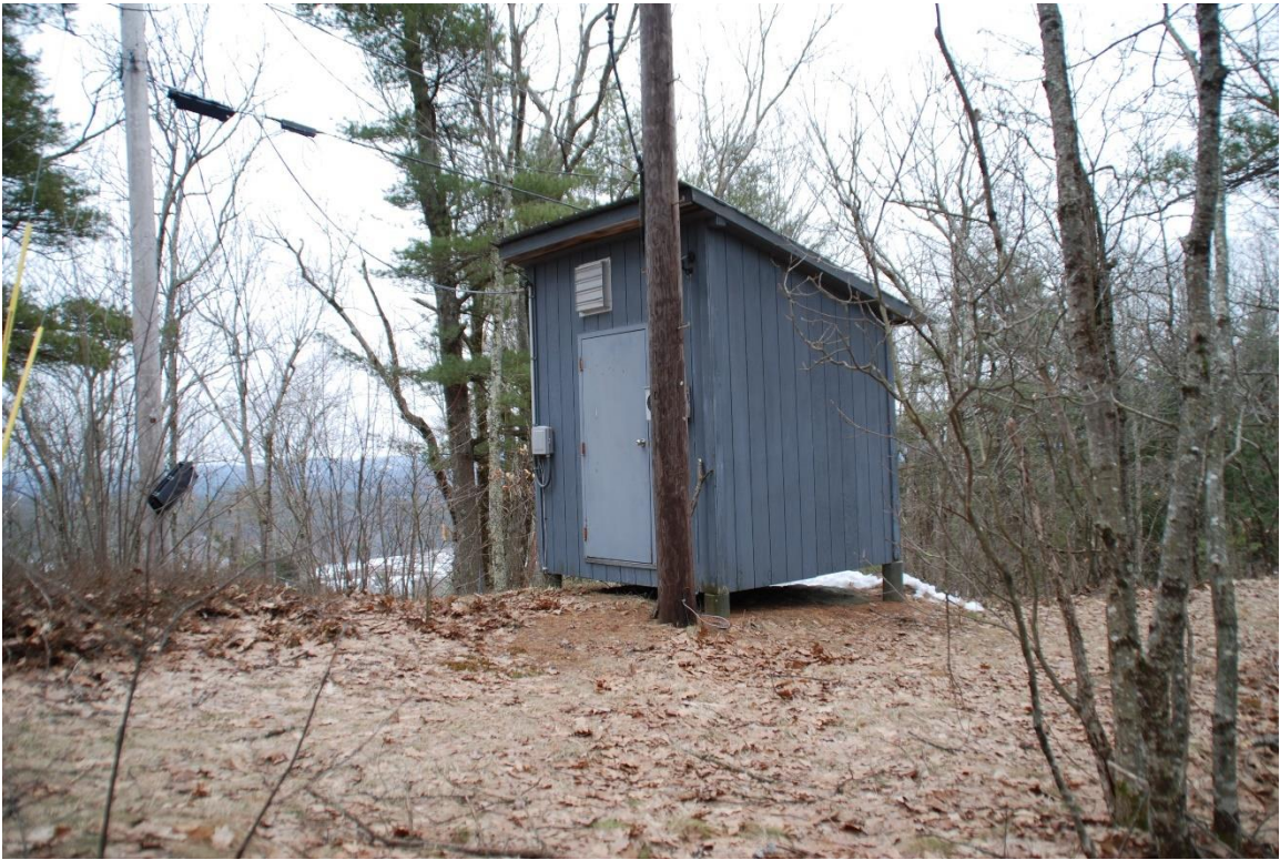
Photo 3. View south of the TDS building where the utilities will lead to the site.
