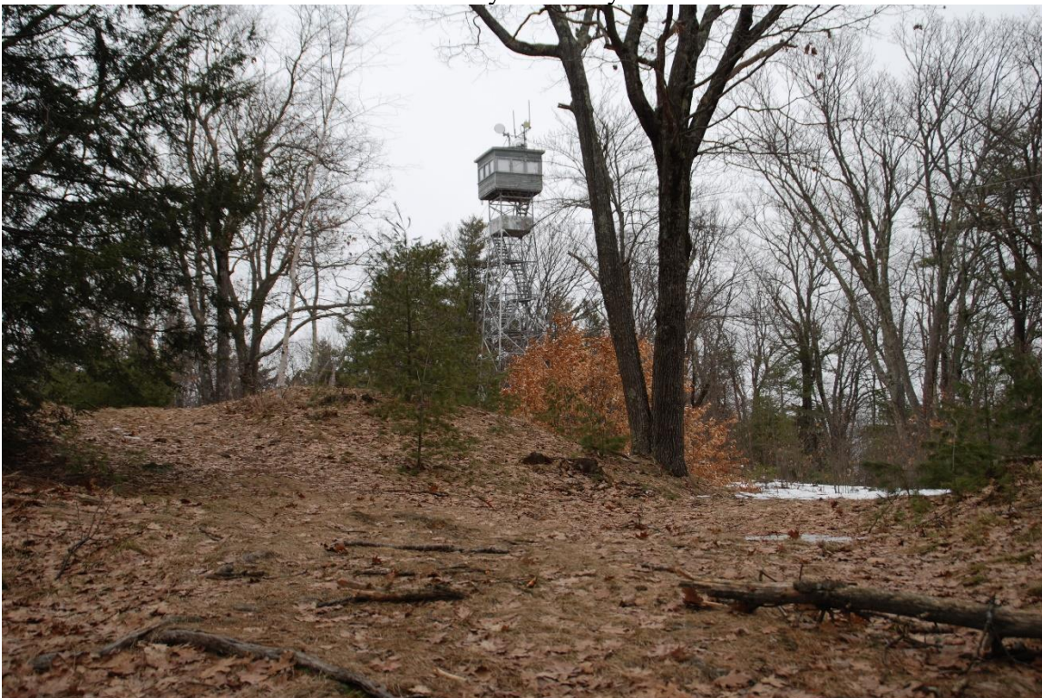
Photo 2. View northeast of the Craney Hill Fire Tower from the access road.
