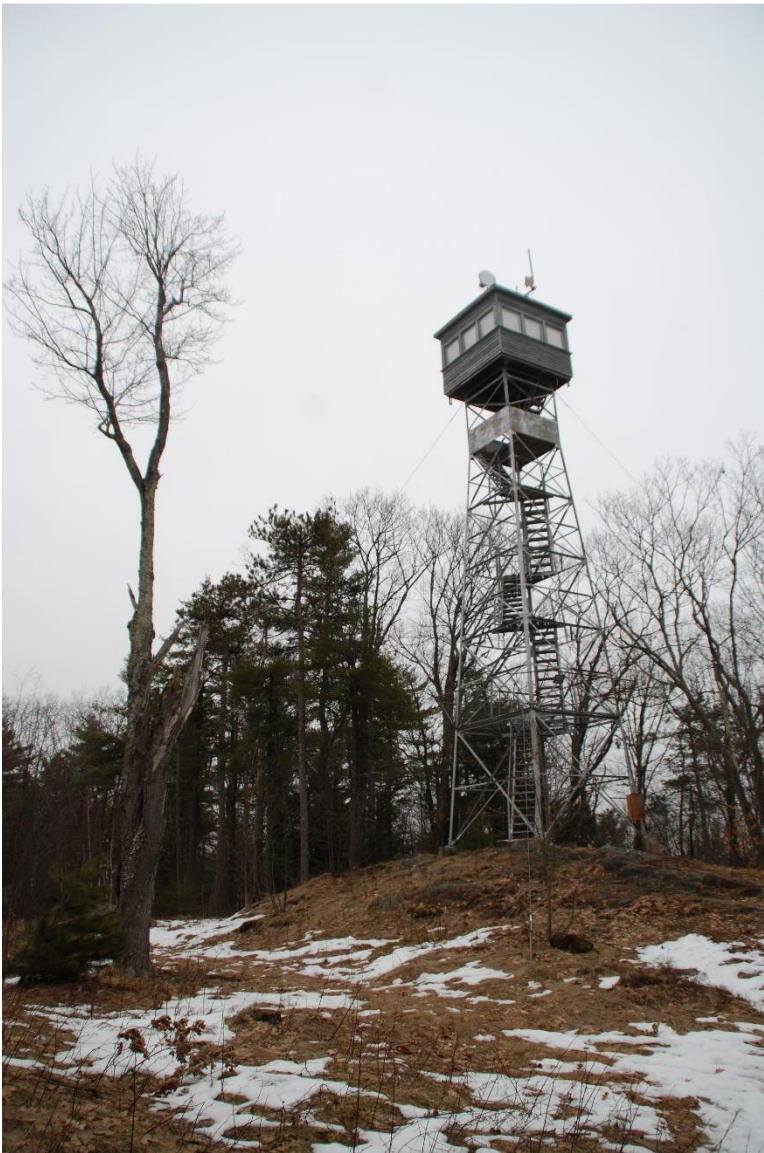
Photo 5. View east of the Craney Hill Fire Tower. The telecommunications tower will be located to the left of the fire tower, beyond the closer pine trees.
