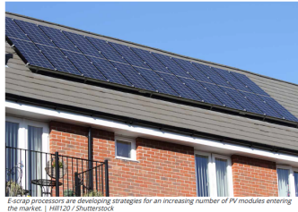
Processing solar panels and developing strategies for an increasing number of PV modules entering the market. | Hill20 / Shutterstock
