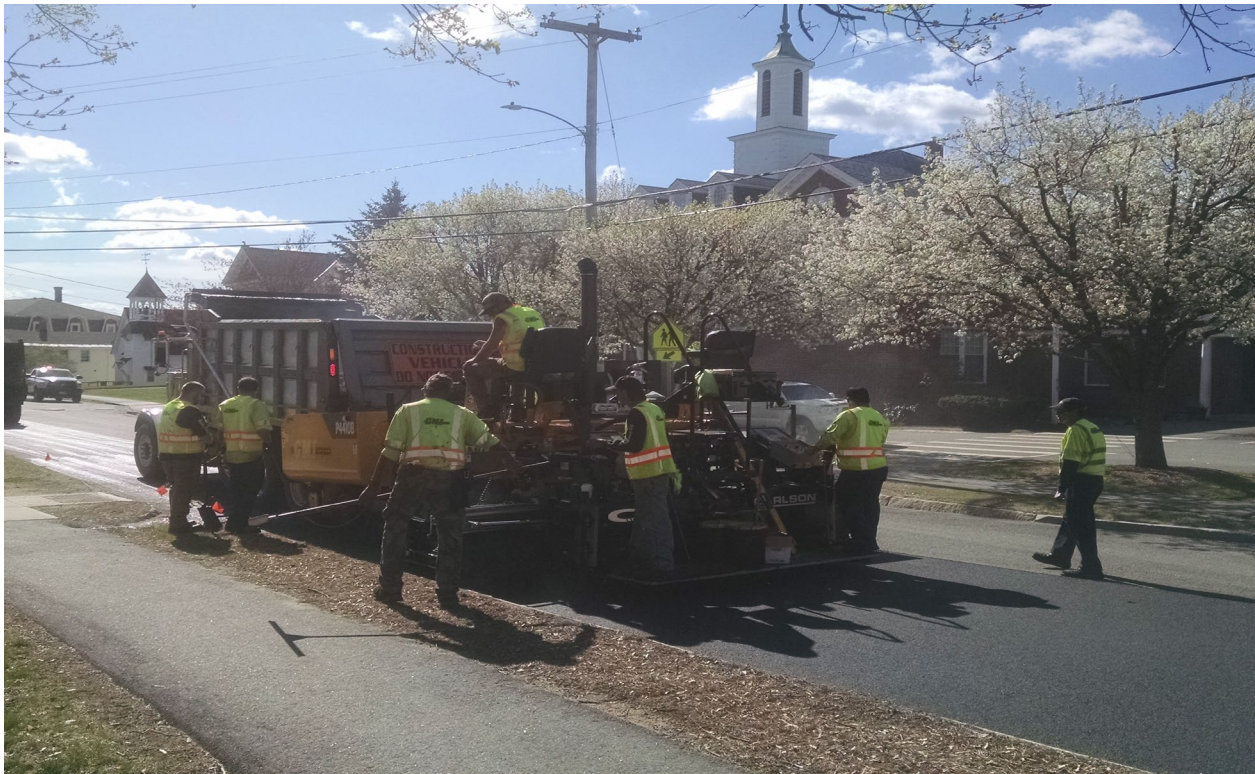
Western Ave. Paving
