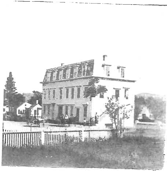
Childs Block, formerly the "Tin Shop", house and barn adjacent
