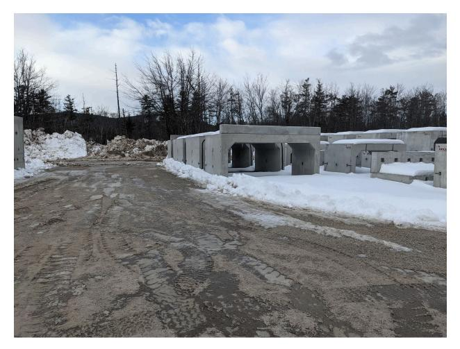
This is a snapshot of the new Bottomless Culvert which will be installed under Liberty Hill Road this spring by Hall Construction.
