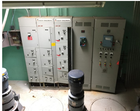
Main control panel in the dry well of the pump station after the water was pumped out. Our pump motors are in the foreground. Everything you see here was completely submerged.
