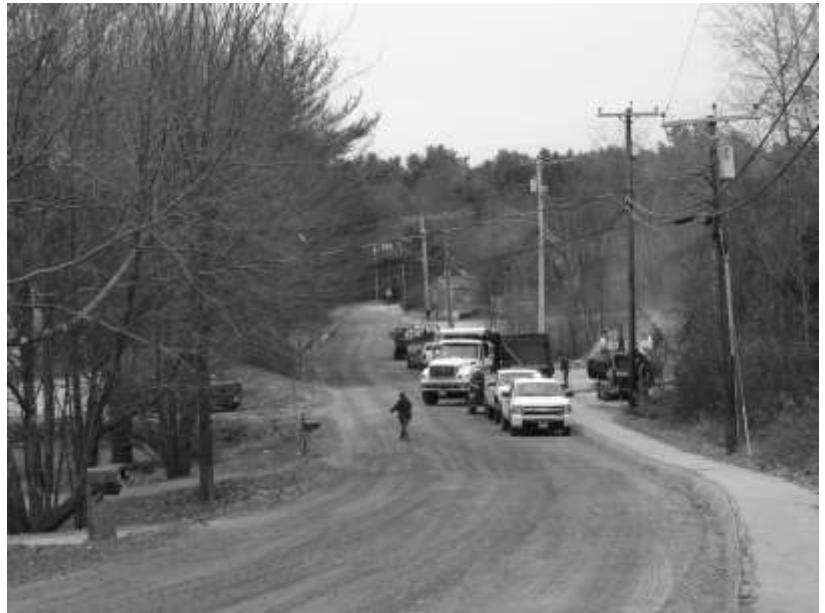
ABOVE: The pavement was reclaimed along Western Avenue in 2012, after the Water Department finished laying new water main pipe.
