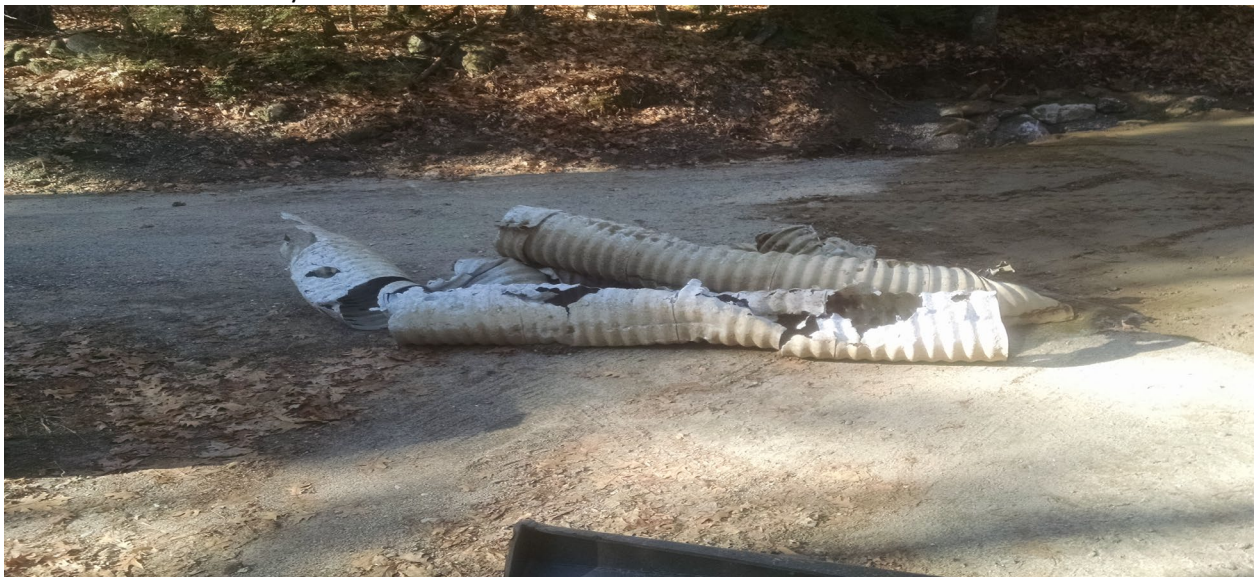
Old aluminum culvert removed from Peasley Road
