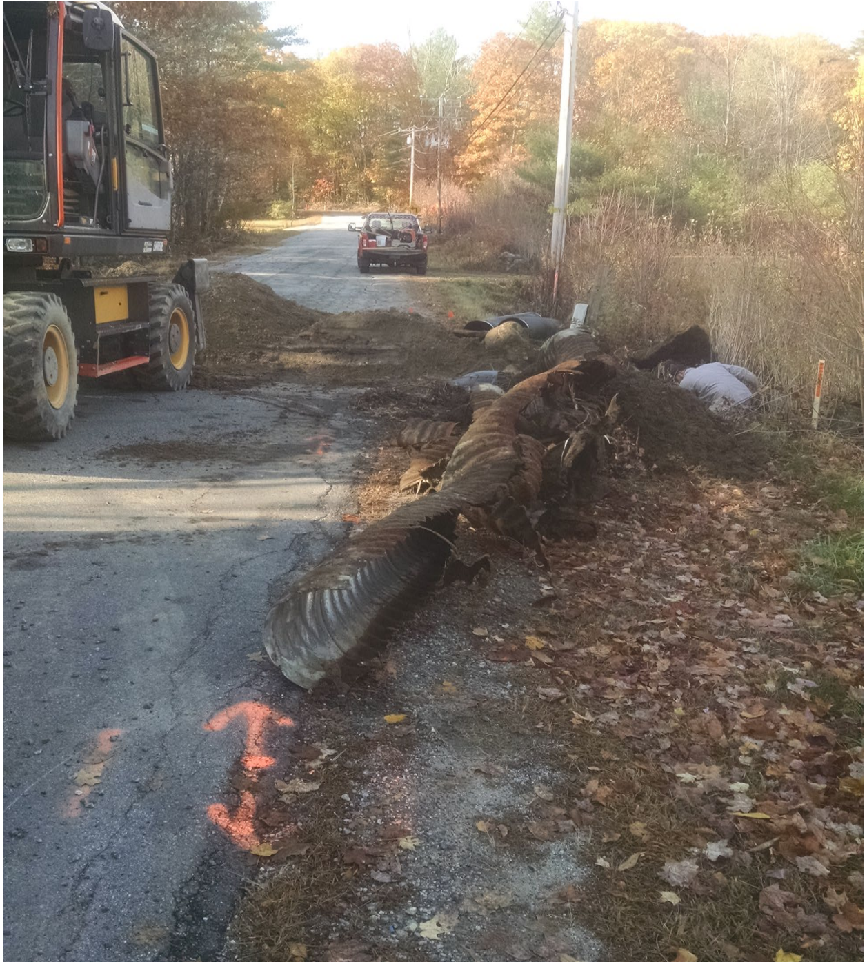
15 inch culvert replaced on Old Hillsborough Rd.
