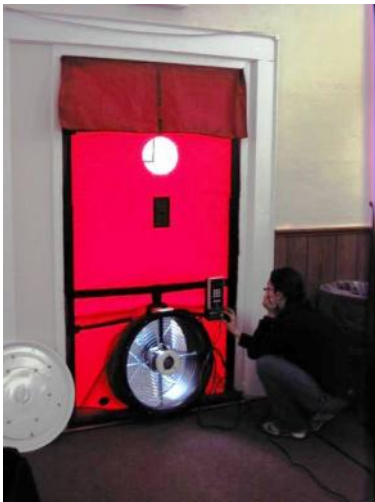
Blower door testing in progress at the Community Center
